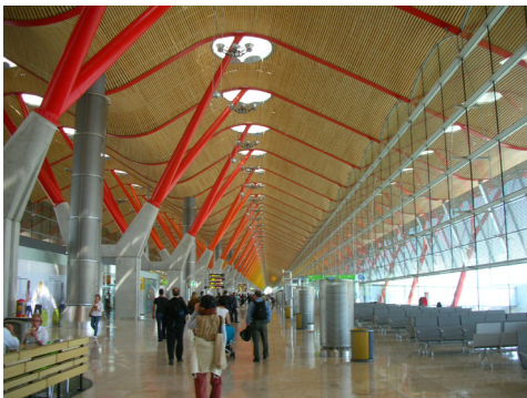
Figura 12: Richard Rogers, Adolfo Suárez Madrid-Barajas Airport Terminal 4, Madrid, 1997-2005
